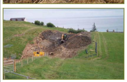
At Sandend last summer, 500 metres of pipe was laid from the village uphill to a new £1 million sewer treatment plant with gravity feed back out to sea.
